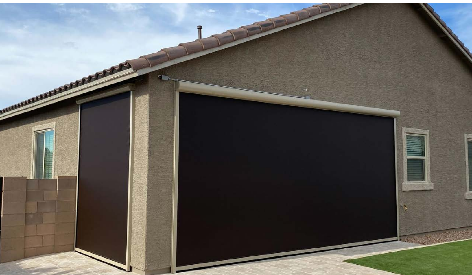
Storm Rail installed by Sonoran Retractable
