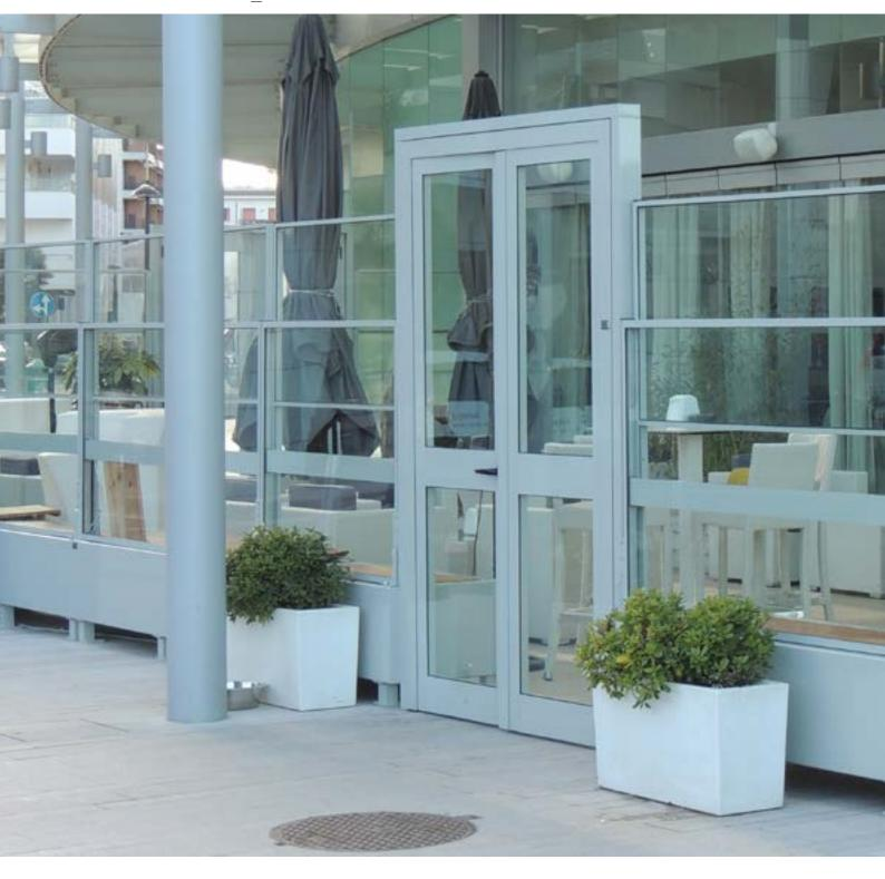
The doors have been designed to provide protection from water and wind. They are made from extruded aluminum alloy profiles (EN-AW 6060-T6) and 4 + 4 pvd 0.76 safety and shatterproof laminated glass in accordance with UNI 7697 2014. Doors are available in either one or two door versions.
